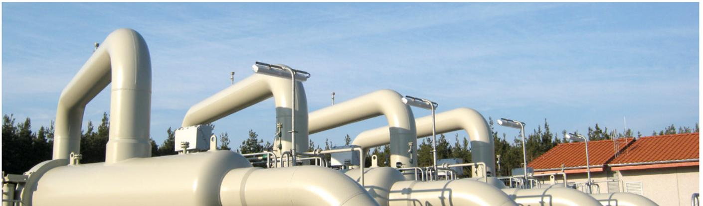
At the Radeland 2 compressor station, natural gas from the incoming pipelines is compressed to compensate for pressure losses. The gas can then be transported onward with the required pressure to the west via the JAGAL pipeline or toward the Czech Republic via EUGAL.
